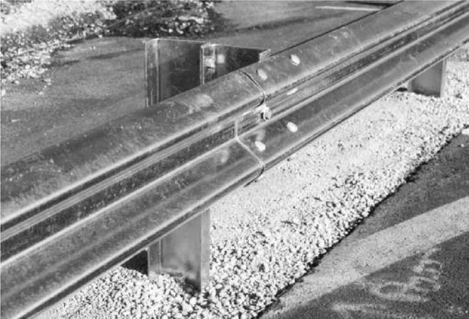
*Figure 4: Strong post W-beam barriers with steel posts and blockouts.*
