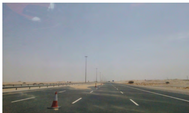
Figure 10. Sand accumulation with existing two-row steel W-beam barriers
