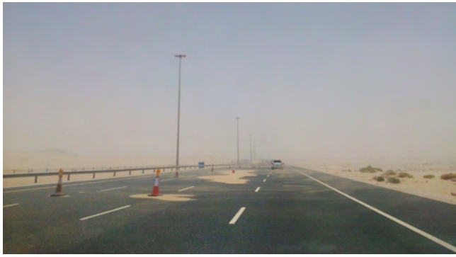
Figure 11. Sand accumulation with a split wire rope and steel W-beam barrier configuration
