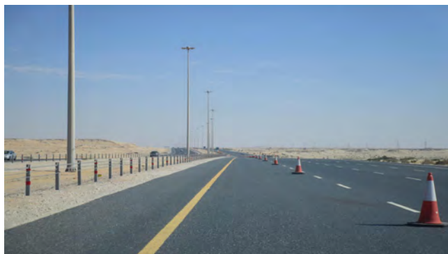
Figure 8. Wire rope barrier installation (August 2015)
