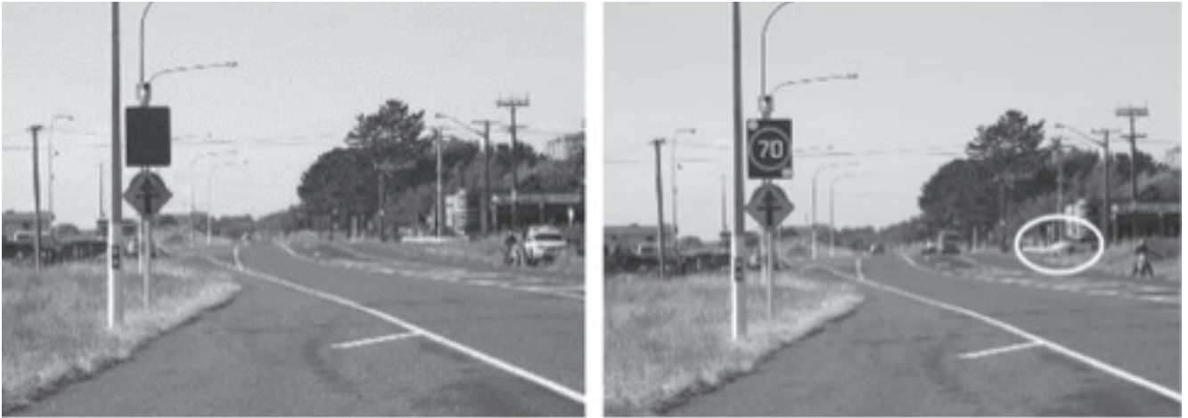
Figure 3. The RIAWS in operation at Himatangi (side-road vehicle is shown in the circle)
