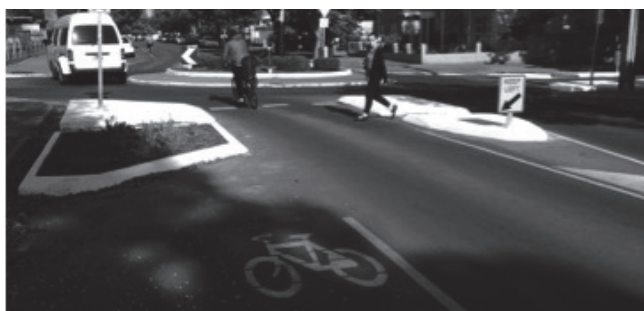
Figure 5. Tangential roundabout redesigned to radial, Beulah Road, Norwood, SA (source: GTA Consultants)
