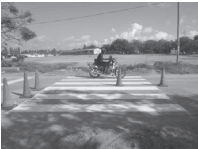
Figure 3. Low cost infrastructure measures – Zebra Crossing
