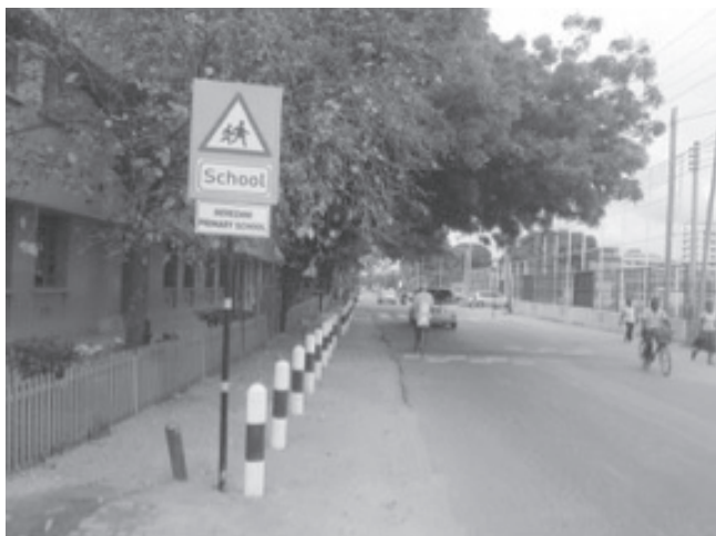
Figure 5. Low cost infrastructure measures – Bollards and Signage
