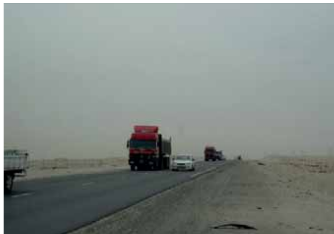
Figure 3. Route 55 before it was upgraded
