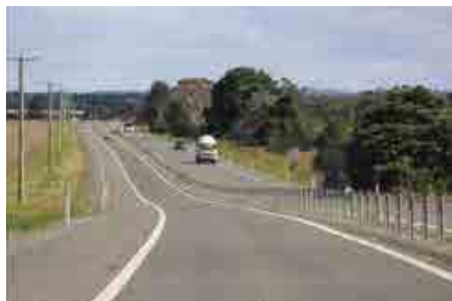
Centre-of-road wire rope barrier
