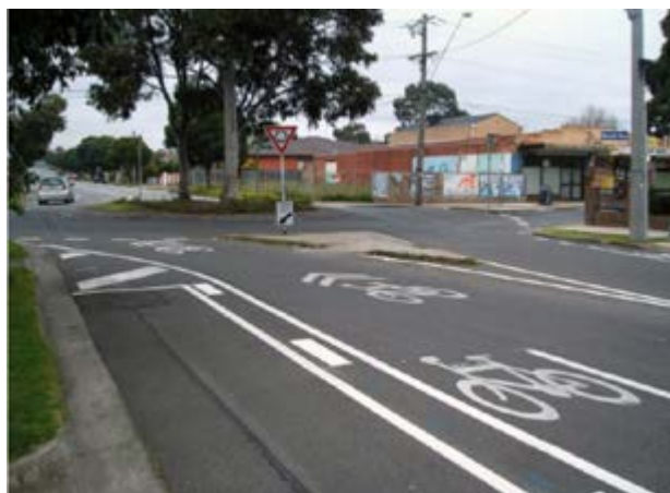
Figure 9. Sharrow road markings
