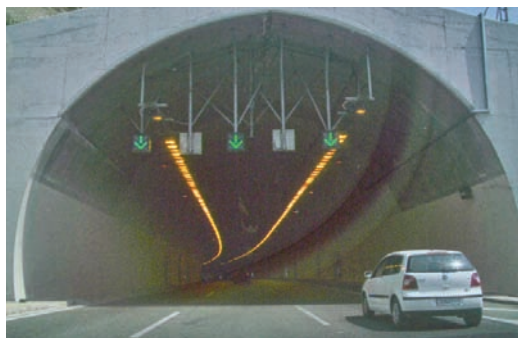
Figures 2 and 3. The luminance contrast can lead to glare (top) or areas to appear darker (bottom) than they really are. The photos illustrate this in a tunnel.
