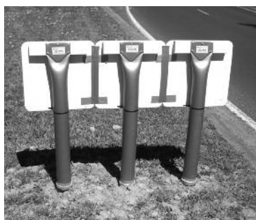
Air-filled plastic posts and sign
