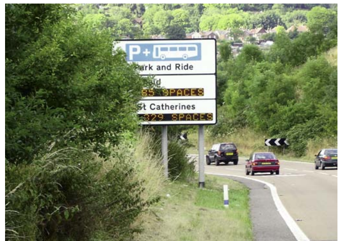
Personally I would be terrified hitting something like this (a heavy VMS sign on rigid steel posts either of which represent an unacceptable risk)
