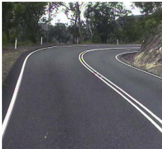
2-star, Gillies Highway Undivided, poor alignment, unsafe roadsides, narrow sealed shoulder width, wide lanes
