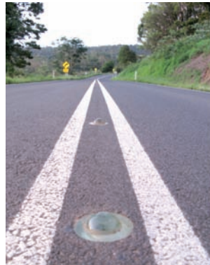
Figure 3. Glass stud delineators installed on a notorious stretch of Kennedy Highway
