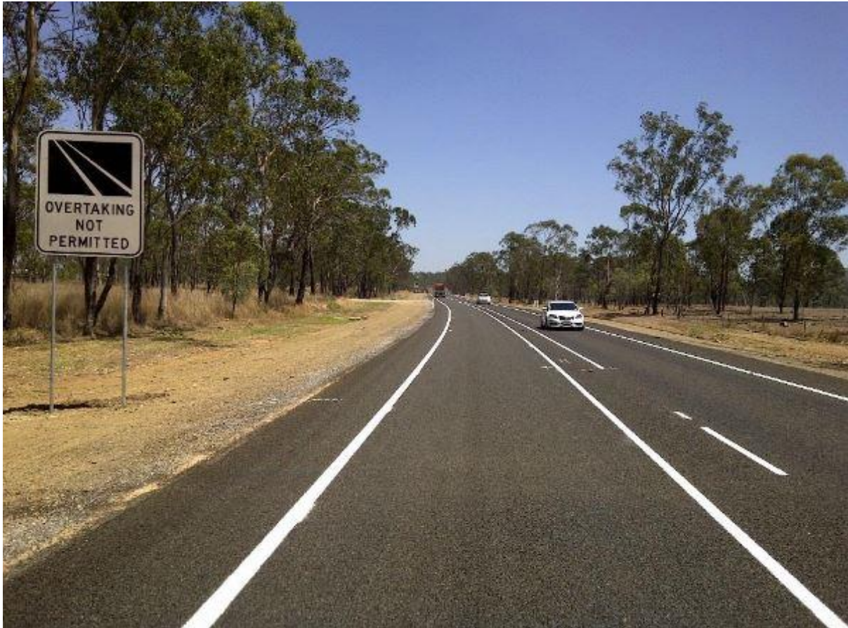
Bruce Highway Centre-Line Widening Treatment
