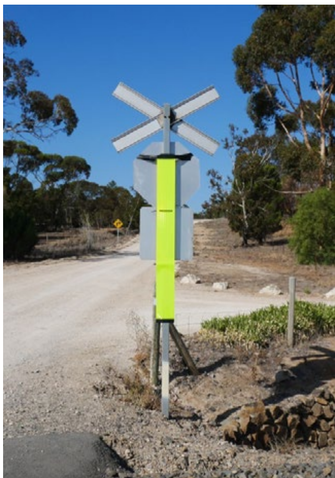
Figure 1. Retro-reflective screen applied to the back of a stop sign
