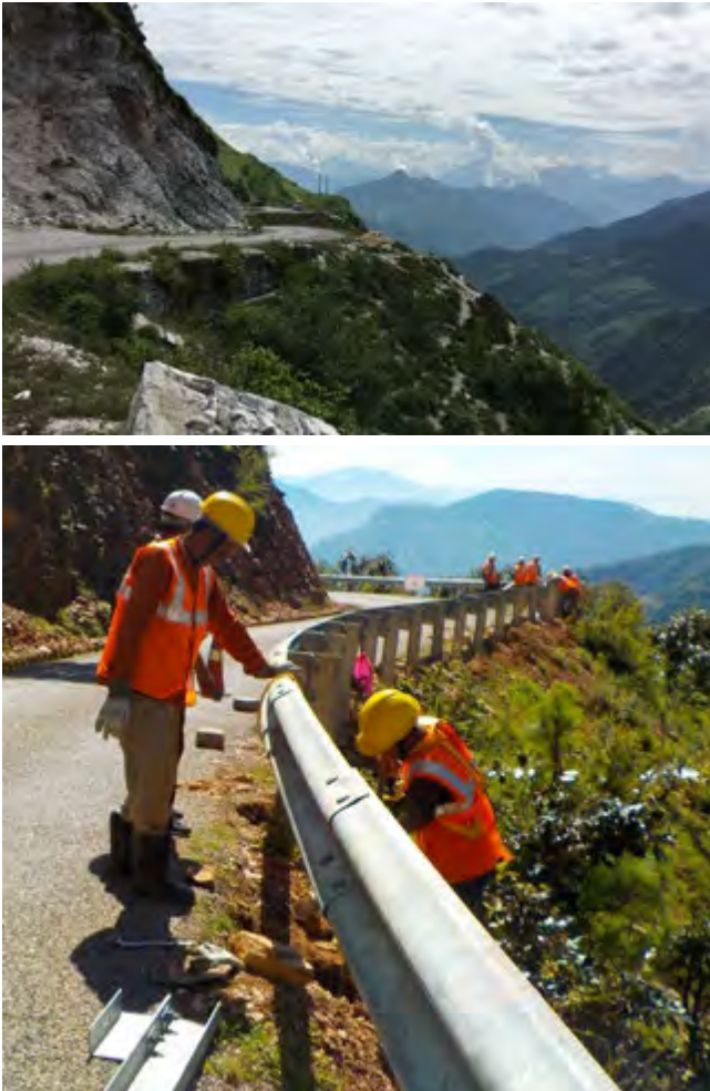
Figure 2. High risk cliff-side roads in western Nepal with and without crash barriers added by GRSF with UK Aid funding (source: Photos by RFS Job)
