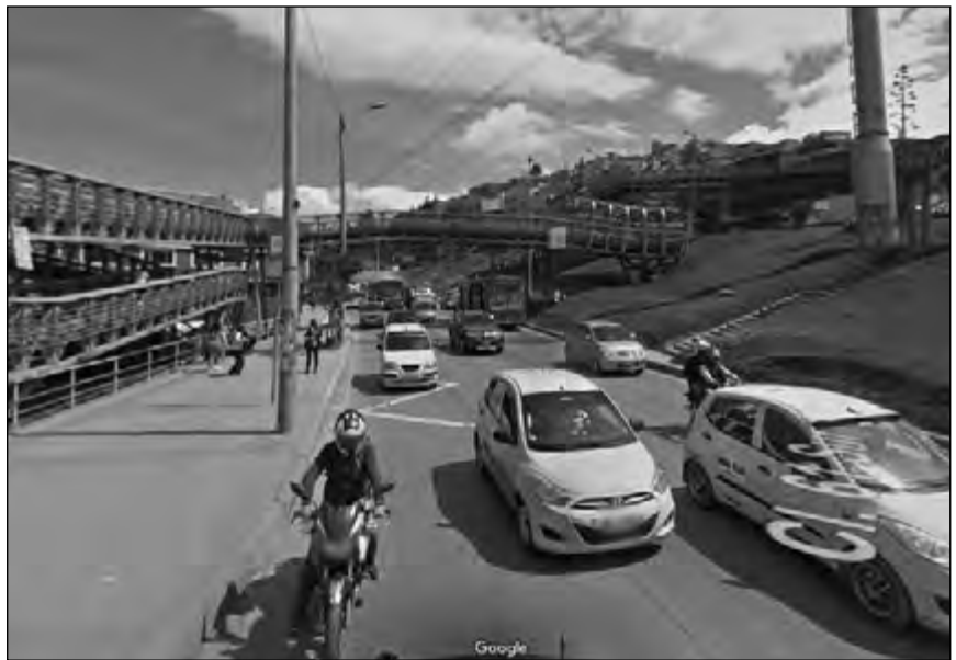
Figure 3. Pedestrian bridge in Bogota.
