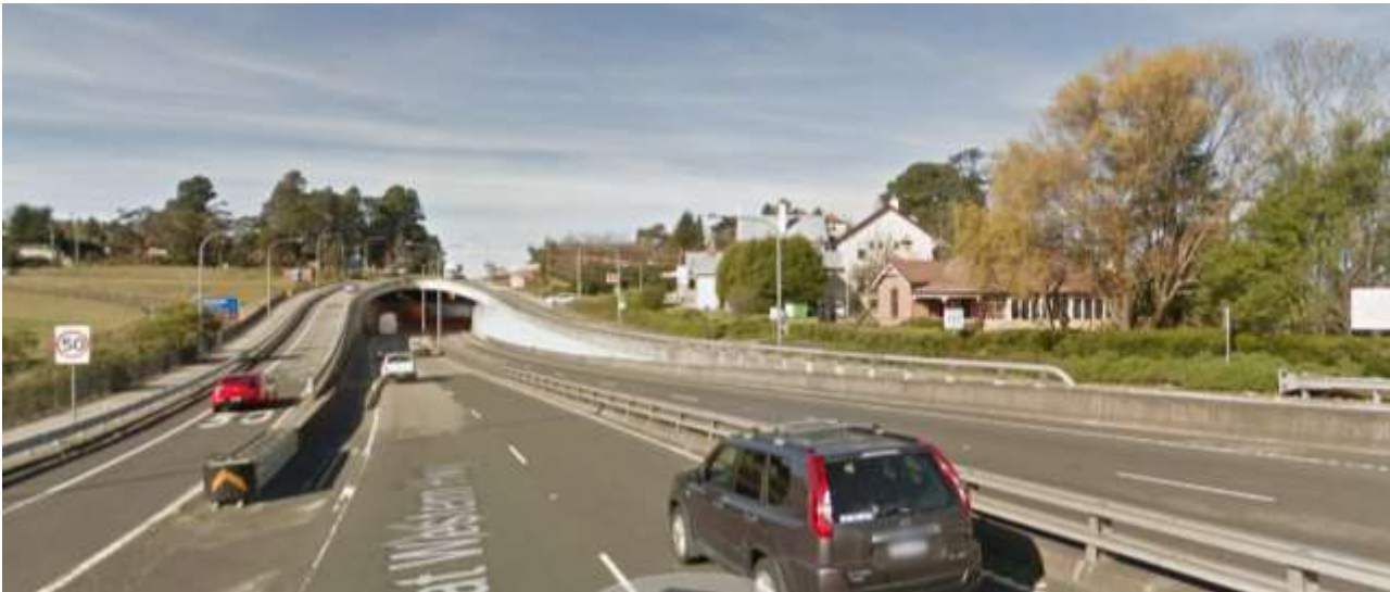
Figure 1a. Great Western Highway showing grade separation at Leura Mall, Leura (Google Maps)
