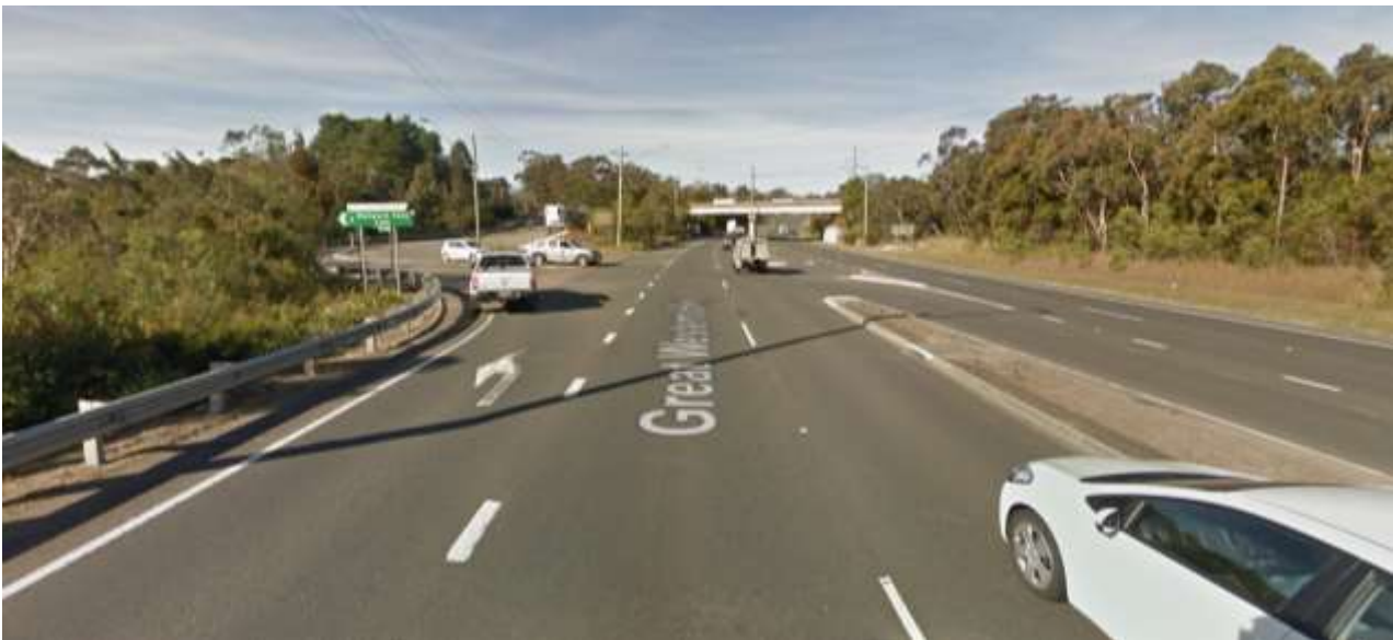
Figure 1b. Great Western Highway at Sinclair Crescent, Wentworth Falls (Google Maps)
