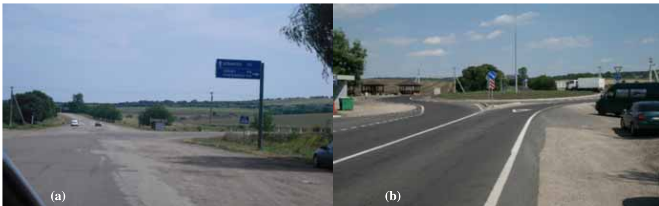
Figure 1. (a) Uncontrolled and unmarked 3-arm intersection “before”; (b) Well-designed and signed roundabout “after”.
