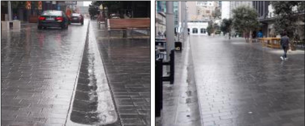
**Figure 4: Drainage Channel Alongside Trafficable Zone – Federal St and Fort St (east)**
