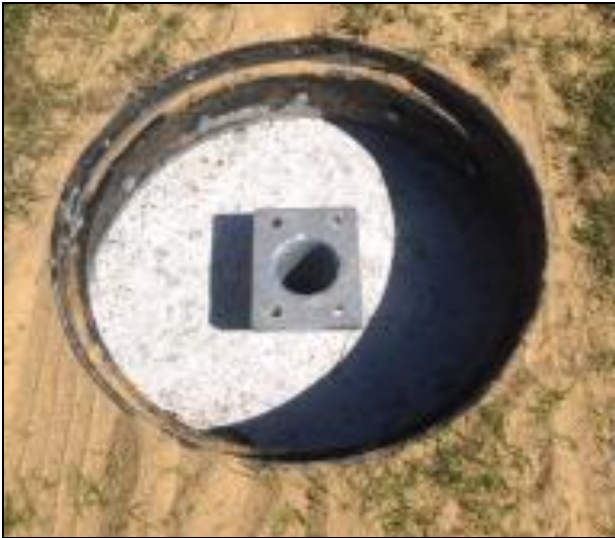
Figure 3.1 – Portable Speed Warning Sign Footing Installed on Council Footpath/Verge
