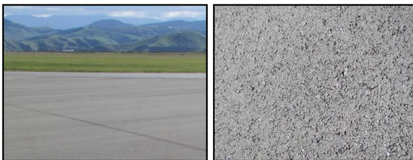
The low macrotexture means this type of surface should not be used in higher speed areas. This particular surface is lightly trafficked which appears to have resulted in the aggregate not being significantly polished to a lower skid resistance.
