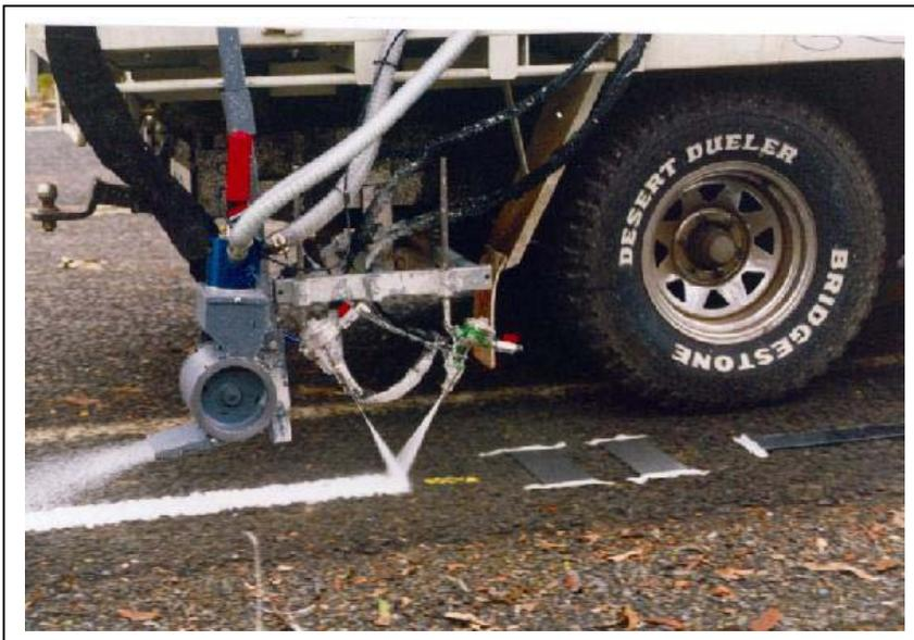
Left: Speedbeader application system. Demonstrating the dual paint gun technique and the static placement of glass beads from the Speedbeader.
