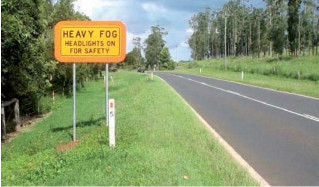
Figure 1. New fog warning signage along a rural highway
