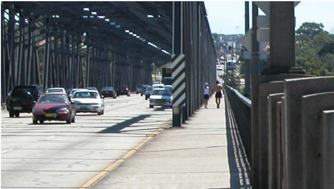
Figure 1: Shared pedestrian cycling pathway on Lane Cove Bridge Sydney. Width of shared space is inadequate for cyclists to pass safely.
