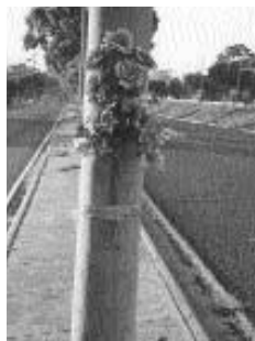
Figure 4: Flowers at scene of concrete pole related vehicle fatality (80 km/hr zone). Note proximity of pole to road.
