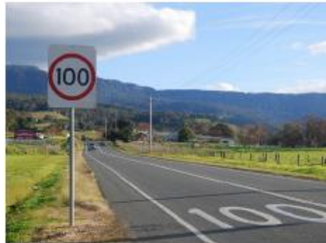
Figure 2: Rural undivided road with sealed pavement greater than 5.6 metres (Source: NSW Speed Zoning Guidelines, page 26)
